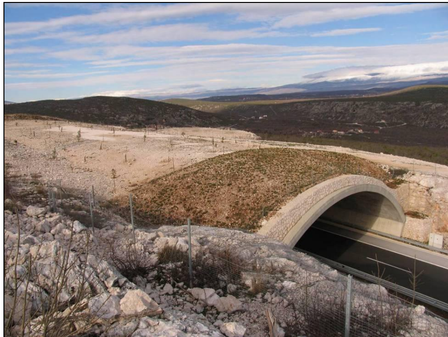
Figure 50. Green bridge Konšćica; one of 5 new green bridges on the highway south of Split (Photo J. Kusak)
