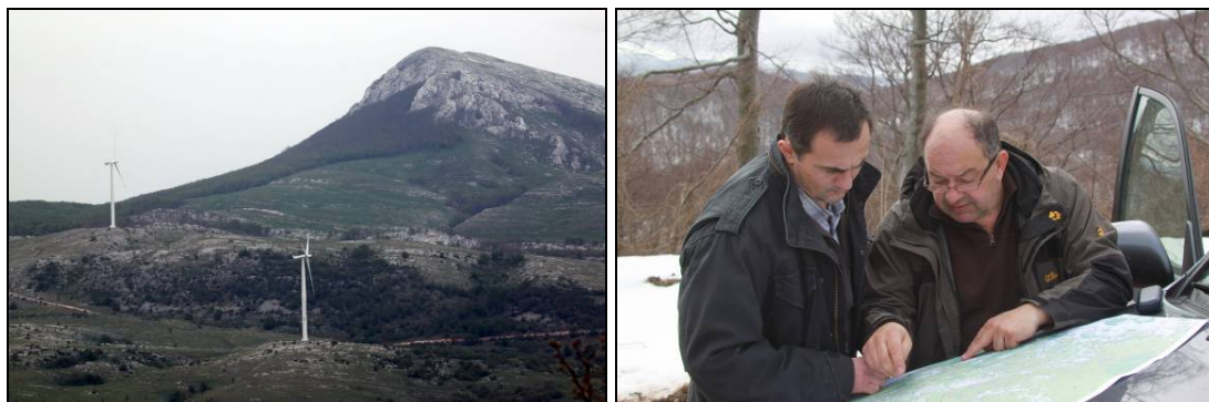
Figure 25 and Figure 26: Wind Park Velika Popina in Southern Lika was already built without considering the presence of wolves in the area. Josip Kusak and Zlatko Prpić (wind parks engineer) during the field evaluation of planned wind park “Senj” on 20.03.2013.
